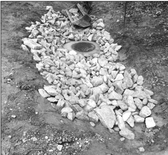
Drainage work on Garrison Ln.
